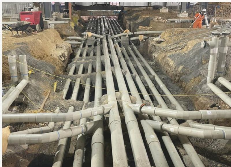
NOV's Fiber Glass Systems has been chosen to provide support for the Fuji Borealis Project. The project, which will feature the Pipex™ Chemsafe PP-H Dual Contained Drainage System, will provide process waste, biowaste, and segregated drainage for a large bio-tech facility. NOV's Fiber Glass Systems' differentiated offerings allow it to meet the specific requirement for biowaste systems containing live pathogens.
