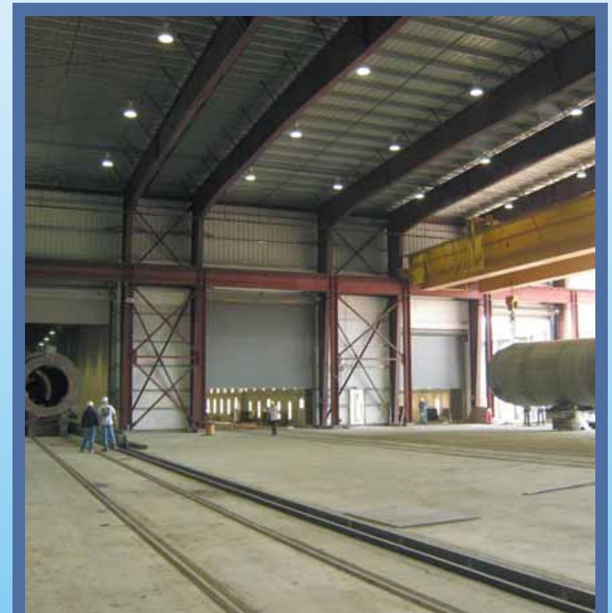
Left to Right: Blast Booth, Paint Booth #3, Paint Booth #2, Metallizing & Paint Booth #1
