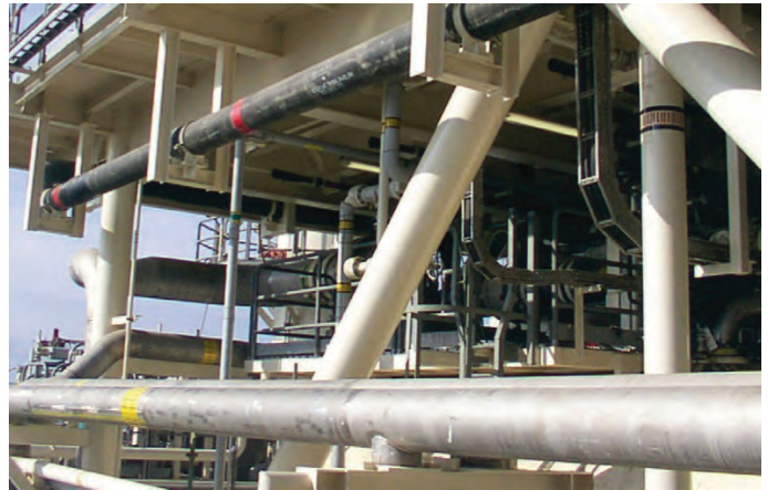
12 in. Bondstrand firewater ring line
