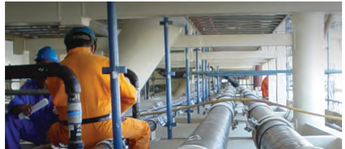
Installation of Bondstrand seawater line
