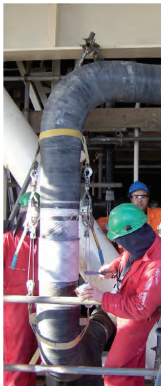
Installation of spool
