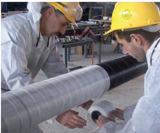
Over-wrapping of fire-protected spool with boat tape
