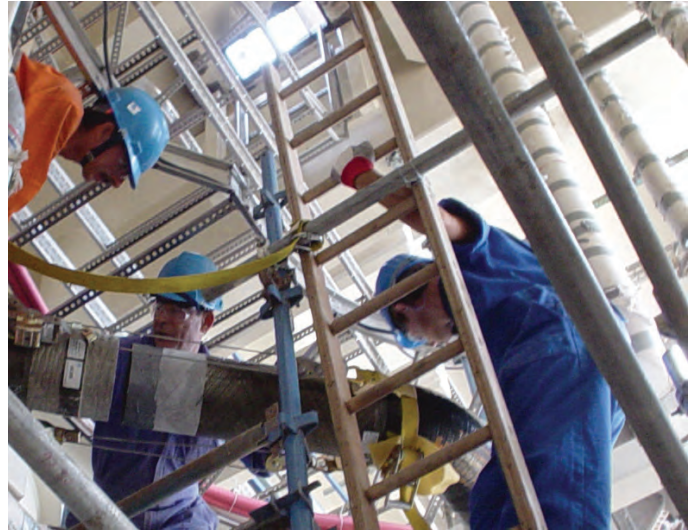
Field joint of pipe spools
