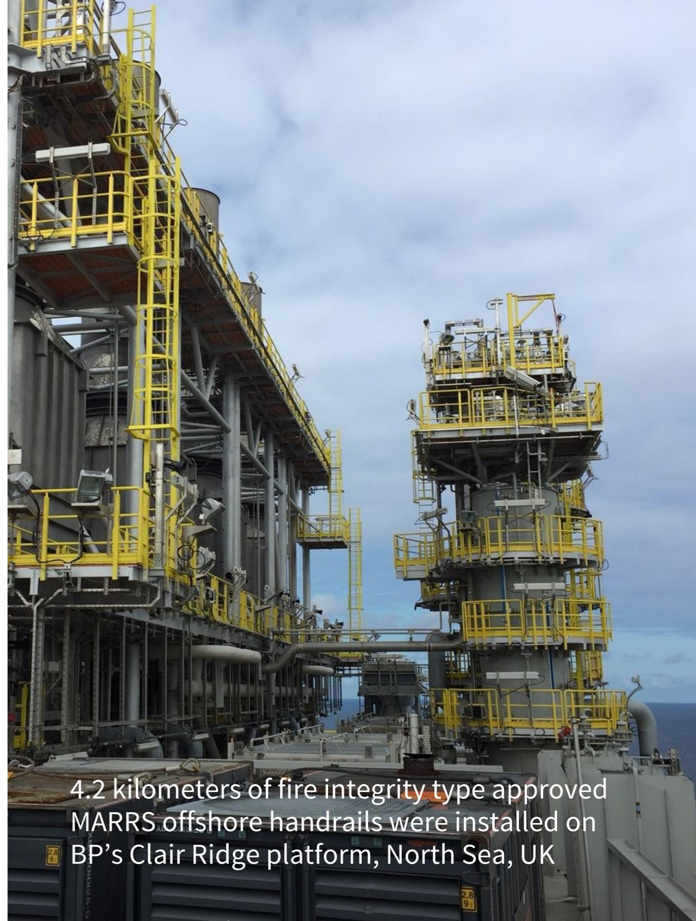
4.2 kilometers of fire integrity type approved MARRS offshore handrails were installed on BP's Clair Ridge platform, North Sea, UK
