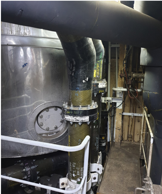
Bondstrand Scrubber Piping on Asuka II. All works were completed in very complicated and confined areas.
