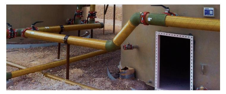
Fiber Glass Systems low pressure line pipe products are very well suited for fittings-intensive piping systems found at tank batteries. Using the same high-grade materials that go into high pressure applications, Red Thread™ HP16 and Bondstrand™ Series 3000A low pressure products utilize a matching taper/taper adhesively bonded joint and provide the features needed for a fast, easy, long-lasting system.
