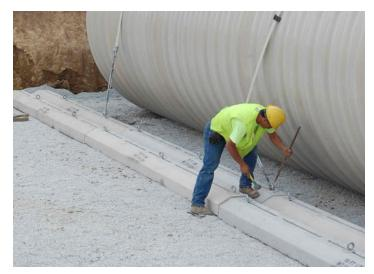
Fiber Glass Systems deadmen include adjustable anchor points for easy positioning and installation.
