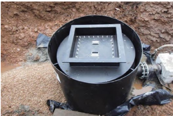
Siltpit with sealed air tight bolted cover and Siltpit with sump recess shuttering to accept concrete surround
