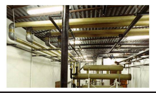
Application: Transfer of sub-zero (-22°F to -40°F) saturated calcium chloride brine solution from refrigeration units to product mold machines to a holding tank for rechilling.
