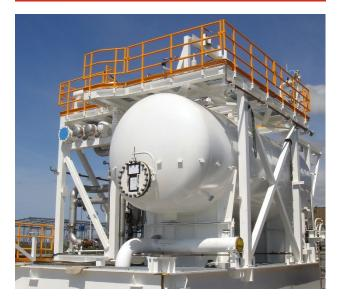
**Customer/End User:** Amerada/Hess **Solution:** Skidded produced water degasser with gas flotation and oil skimming features.
