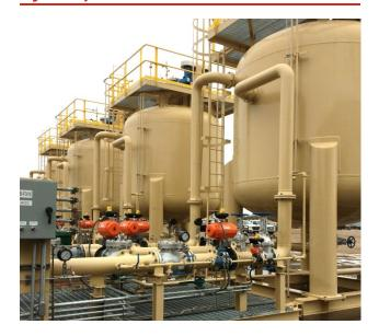
Customer/End User: Worley Parsons/Chevron Solution: Water plant expansion with 4 off 12 ft diameter nutshell filters, each designed to handle 50,000 BWPD.
