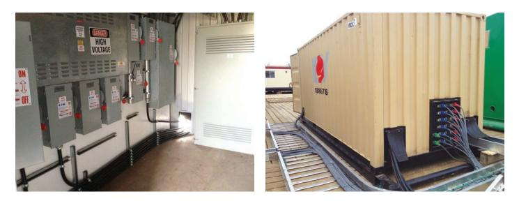
Electrical distribution can be customized for your site specific requirements ranging from a simple stand-alone pedestal to a 20ft. enclosure with a 2,000 Amp automatic transfer switch, transformers and multiple breakers / disconnects to meet your application.
