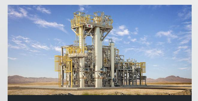
This year, NOV secured a contract to provide a deoxygenation and dehydration package for a green hydrogen project being developed in Australia by an integrated energy and metals company. This is NOV's first order for hydrogen treatment technologies, which was received after completing an extensive engineering process study for treating hydrogen gas downstream from an electrolyzer.
