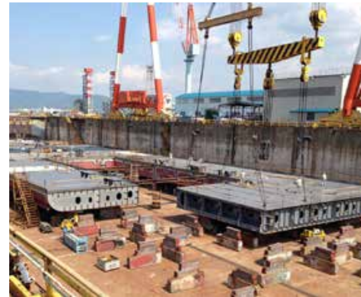
Qdrill under construction at Ecovix
