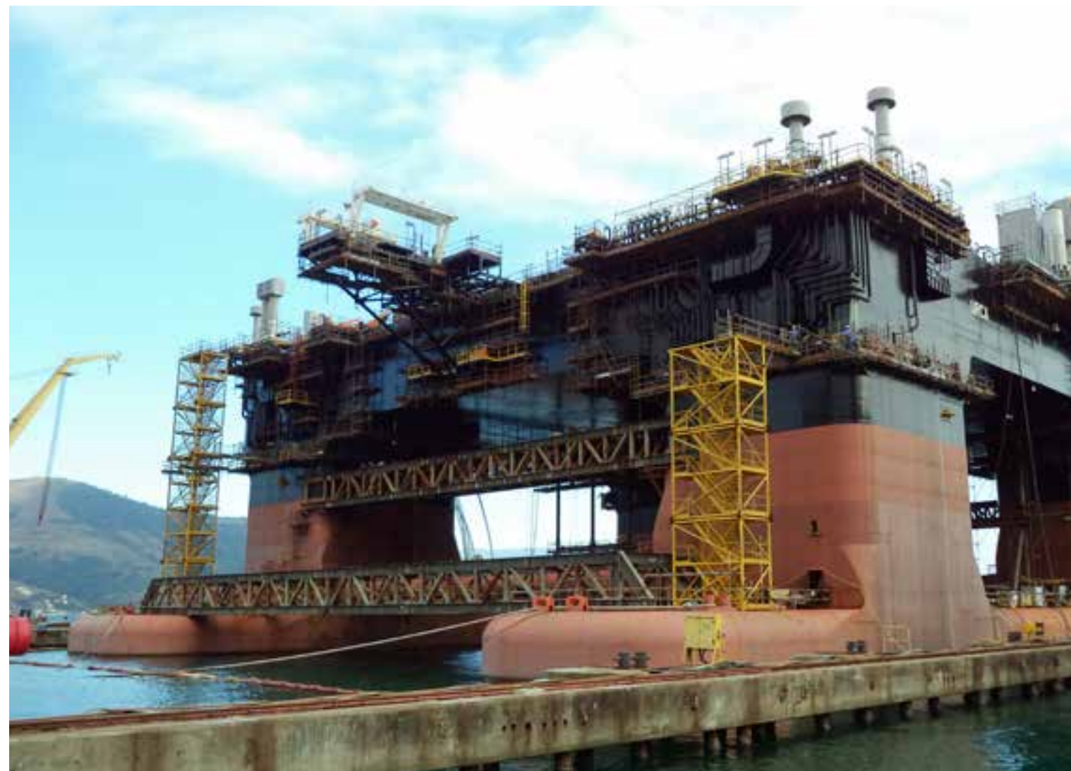
Semi-sub under construction at BrasFels
