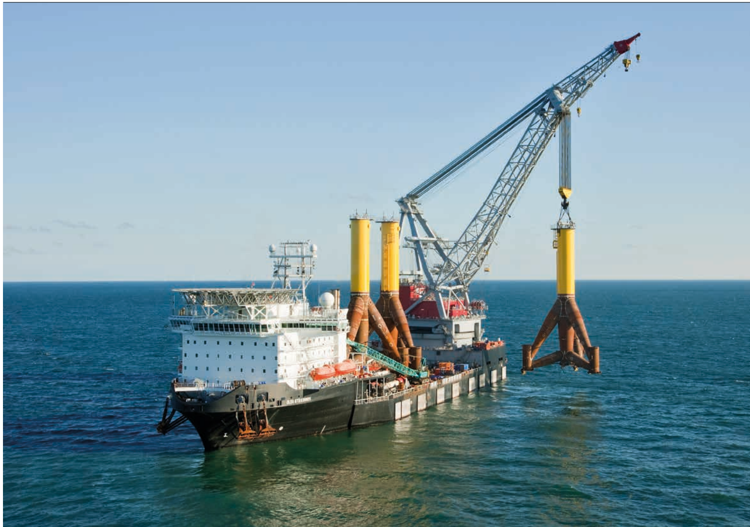
The 5,000 tonne crane vessel Oleg Strashnov installing wind turbine foundation tripods at Borkum West II Windfarm. The vessel as well as Oleg Strashnov's 5,000 tonne and Stanislav Yudin's 2,500 tonne cranes are GustoMSC designs.
