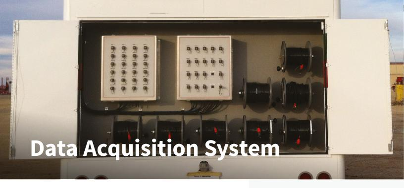
Our data acquisition controls system (DAS) is our hardware-based acquisition system to bring in raw signal data, scale, and display actual values.
