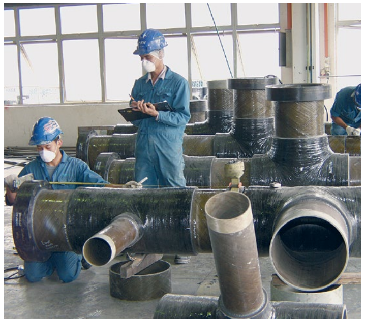
Prefabrication of custom made fiberglass spools
