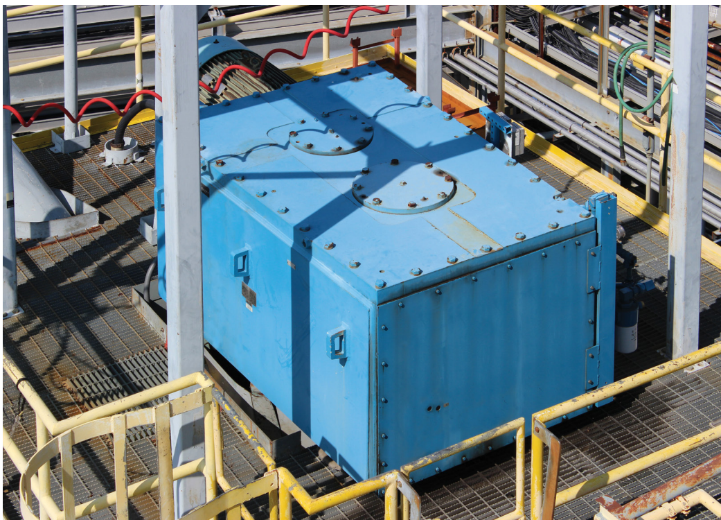
Installed Chemineer HT agitator
