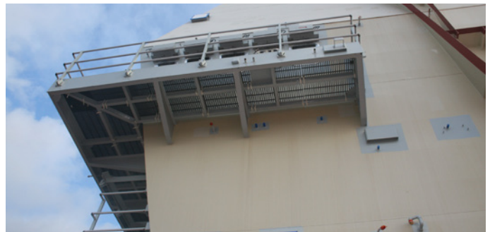
FRP structures installed
