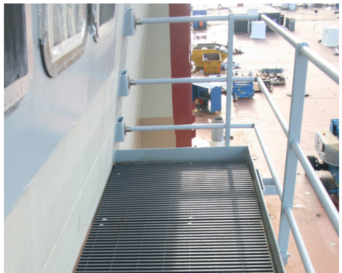
FRP structures installed
