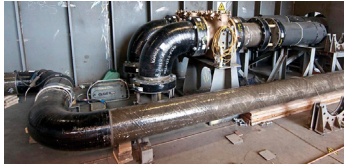
Bondstrand GRE pipe installed on QEC
