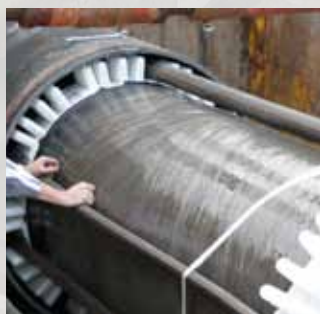
DN900 Bondstrand in DN 1200 casing
