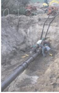
aid of laser-guided excavators. This approach of trench preparation often resulted in trench depths of more than 5 meters.
