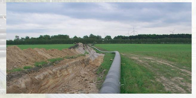
In 2001, NOV Fiber Glass Systems B.V. secured the contract for an 18 inch GRE brine transport line with a working pressure of 20 bar with a total length of 54 km. Leading energy supply company EWE (Elbe Weser Ems) planned to create four caverns, at a depth of 1200 meters, 450 meters high and 100 meters in diameter, with a volume up to 700.000 m<sup>3</sup> each in the underground salt layers of Rüdersdorf, located some 30 km east of Berlin. The caverns were created for storage of natural gas.
