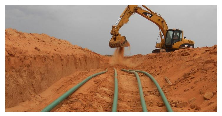
Fiberspar LinePipe is a spoolable glass-reinforced epoxy pipe which has achieved widespread preference over welded steel pipelines for in-field gathering and injection applications. Already widely used in oil and gas fields throughout North America, it has now been successfully installed for a major operator in Australia, creating new opportunities for efficiency and cost savings in the region.
