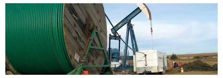
Spoolable, composite LinePipe provides an exceptionally cost-effective way to remediate old or damaged pipelines with minimal excavation or surface disturbance. And now, NOV Fiber Glass Systems is the only company with the full breadth of installation processes for remediation available in-house.
