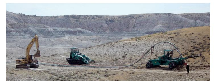
Plowing can be a fast and low-cost installation method for Fiberspar LinePipe. Using a high-capacity plow to install Fiberspar LinePipe can be an innovative and cost-effective option.
