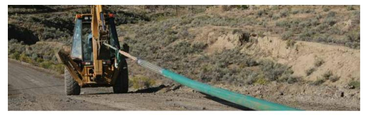
Since Fiberspar LinePipe is laid continuously, installation times as low as one-third of that required for steel pipe have been documented. Often, installation is so rapid that extra ditching equipment actually has been delivered on-site to maintain pace with the expertly trained and highly experienced NOV Fiber Glass Systems crews. Not only are installation costs slashed compared to steel pipe, but Fiberspar LinePipe also effectively eliminates the subsequent costs associated with corrosion.
