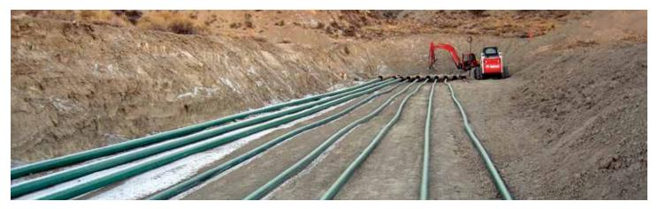
Whether your application is for a new sweet/sour oil or gas gathering line, or for a high-pressure water or CO<sub>2</sub> injection system, NOV Fiber Glass Systems spoolable pipeline system is your best performing and lowest cost alternative. No other spoolable pipeline supplier offers the range of products, diameters, pressure ratings, temperature tolerances and terrain-specific installation methods—open ditch, plowing or remediation—than does NOV Fiber Glass Systems.
