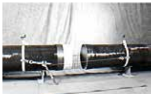
Photo 6 Ratchet-Type Cable Come-Along
