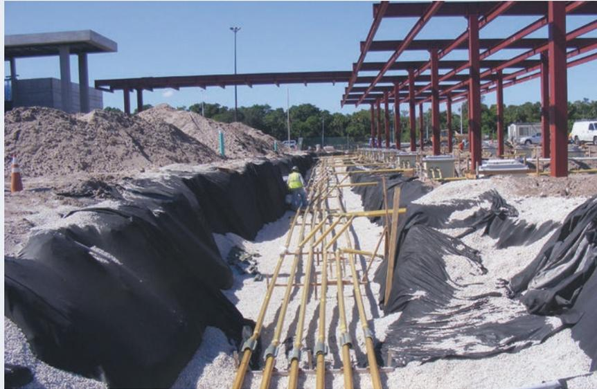
Red Thread IIA pipe was installed at the Pompano Beach Plaza in the 1970's and continued to perform into 2011. When it became necessary to redo and enlarge the rest stop again, the contractor chose the product that had worked for over 30 years.
