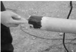
Apply paste to pipe
