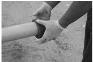
Stab mold onto pipe
