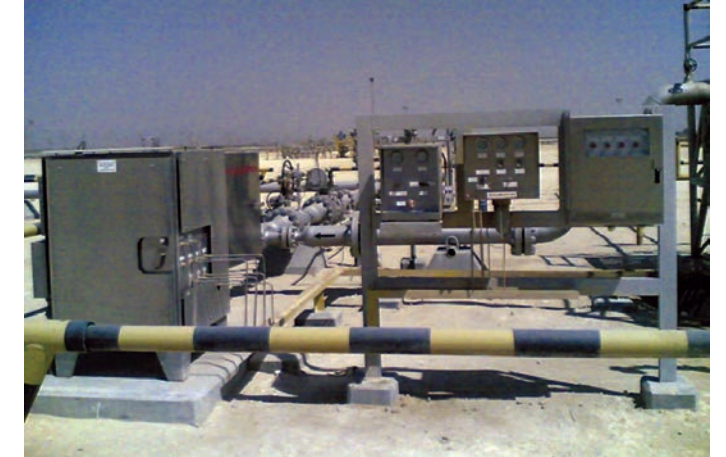
Multi-Well Control Panels
