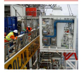
Customer/End User: Aker Solutions/Premier Oil Solution: 35,000 BPD system cleaning produced water to <15 ppm oil. The system is designed for retrofit into the existing platform and consists of booster pumps, deoiling hydrocyclones, and compact flotation units.
