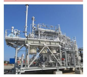
**Customer/End User:** GSP Offshore/BlackSea **Solution:** TEG contactor + TEG regeneration skid 3 m<sup>3</sup>/h. Assembly completed on site, ready for commissioning.
