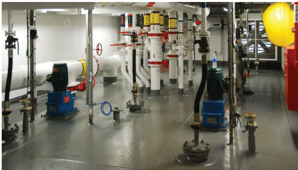
Installed Model 20 agitators on an oil rig
