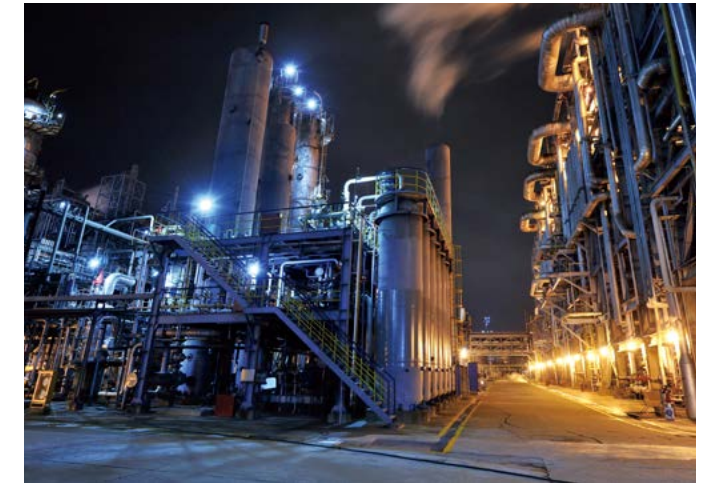
Chemical, Pharmaceutical, Petrochemical
