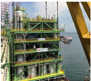
Customer/End User: BWO/Premier Oil Solution: 500 m<sup>3</sup>/h SW, 828 m<sup>3</sup>/h PW. 1758t module (33m x 24m x 24m) consisting of produced water treatment and seawater treatment, combined.
