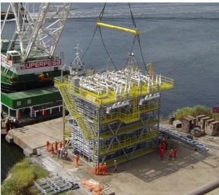
Customer/End User: QGI/Petrobras Solution: 220,000 BPD Module consisting of coarse filters, cartridge filters, SRU, and deaerator (loose).
