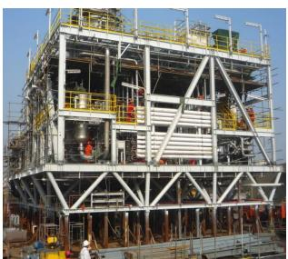
**Customer/End User:** Modec/Petrobras **Solution:** 100,700 BPD module consisting of coarse filters, multimedia and guard filters, deaerator, and SRU.
