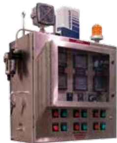
Titan BX Control Panel
